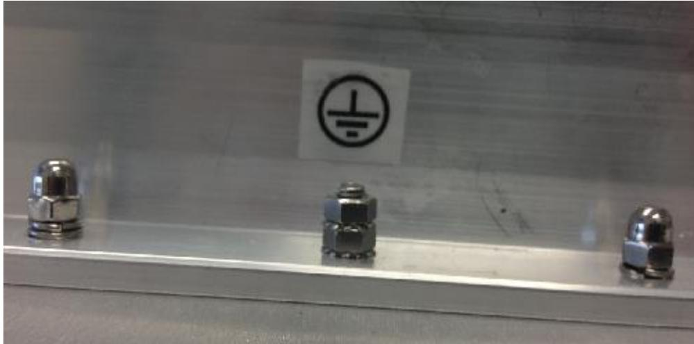
Figure 5-1 – 9502 Protective Earth Grounding
